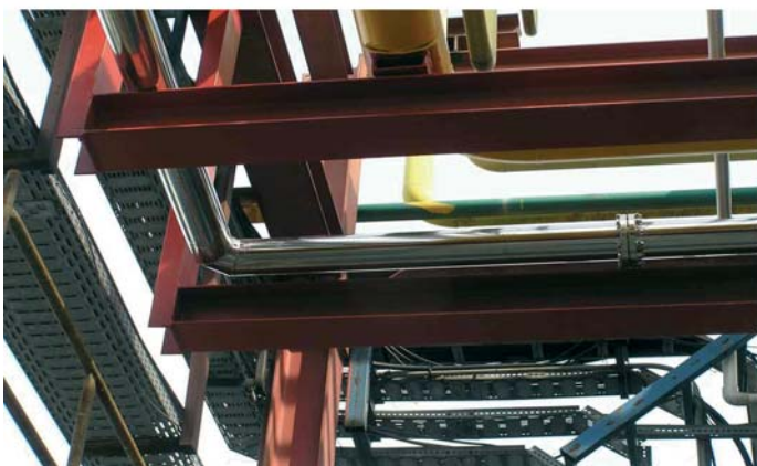
Vacuum Insulated Pipeline for liquid nitrogen
